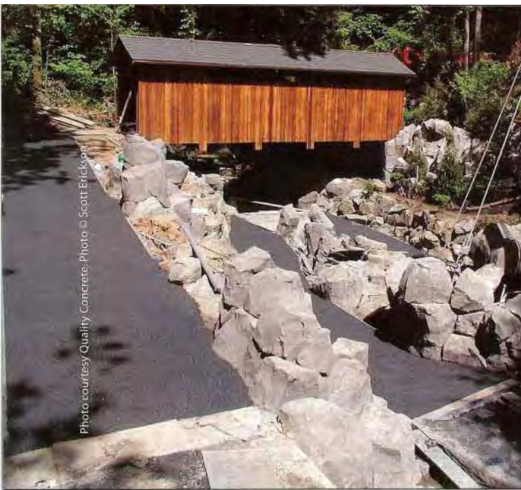
Pedestrian safety at Portland's Oregon Zoo is increased with pervious concrete walkways providing a non-slip surface in all weather conditions without supplemental drainage.
