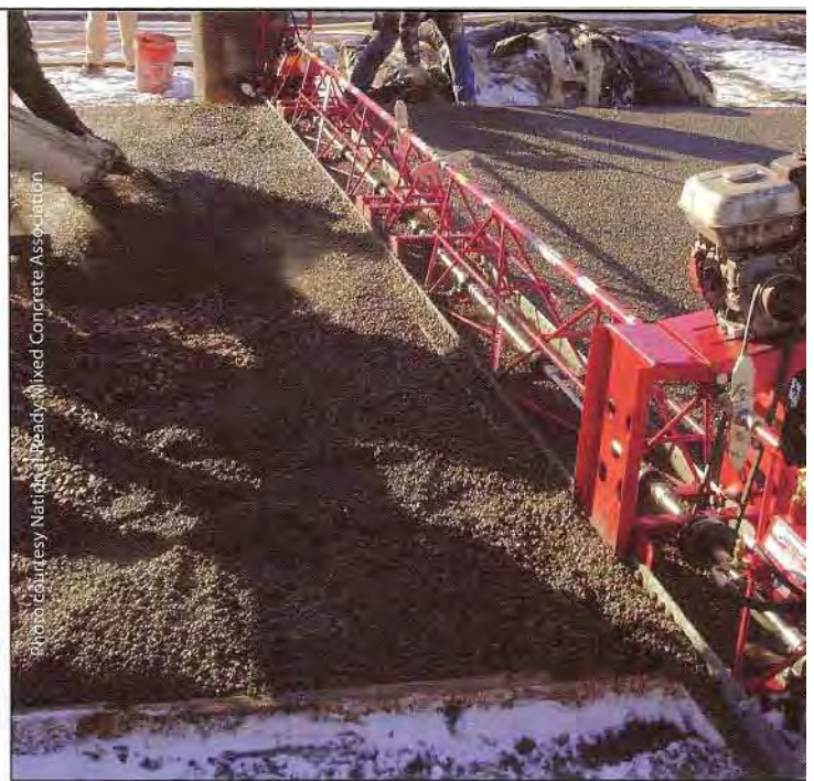
Vibratory screeds are frequently used in the placement of pervious concrete, such as in this Denver, Colorado, Safeway supermarket project.
