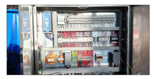
Inside said cabinet, there are the frequency converters for lifting and rotation as well as all accessories.
