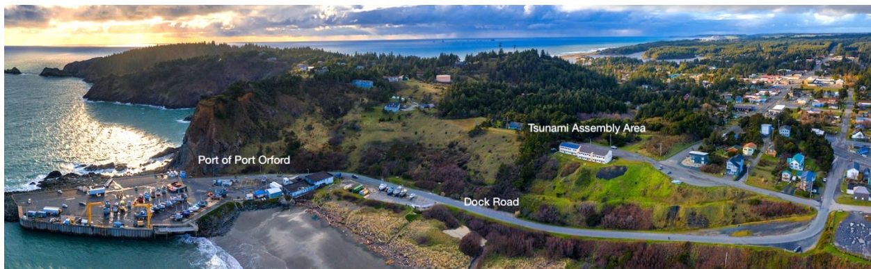
Figure I-13. Port of Port Orford, Aerial View.
