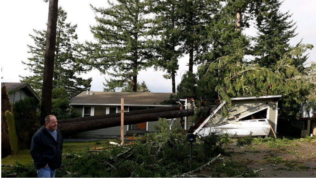
Figure I-54. Residential Windstorm Damage Brookings, 2019
